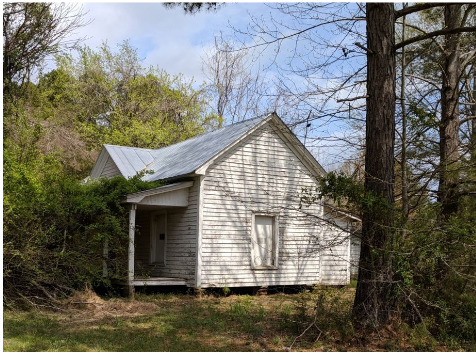
The former Laws family residence (unoccupied)
